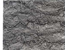
CSP 9 (heavy scarification)
